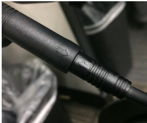
The main connection is shown with both arrows aligned and the wires fully plugged in.
